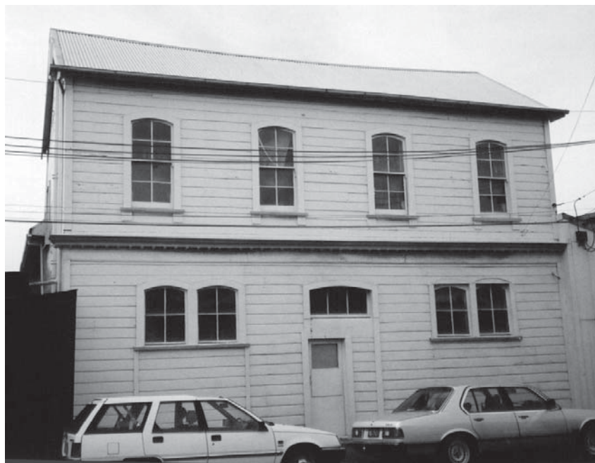
The upper storey segmental arched windows of the Oddfellows Hall show this to be clearly a Victorian-era building. (M. Kelly)
